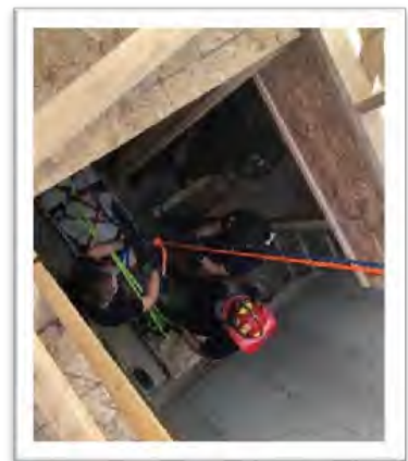
Below Grade Rescue
