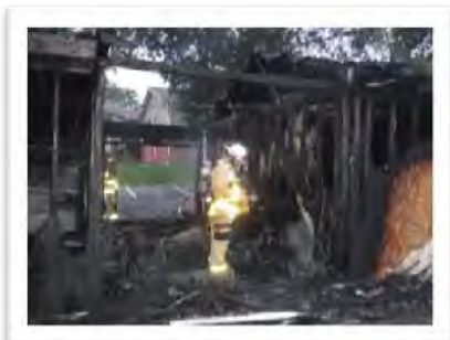
Greenway Cross Structure Fire
