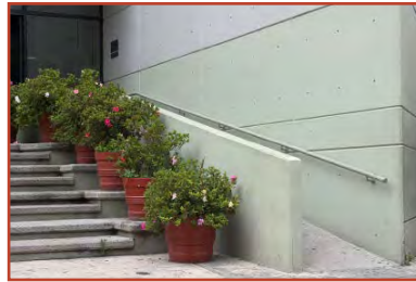
The ADA ramp is incorporated in the stair entrance and meets the needs of all users.
