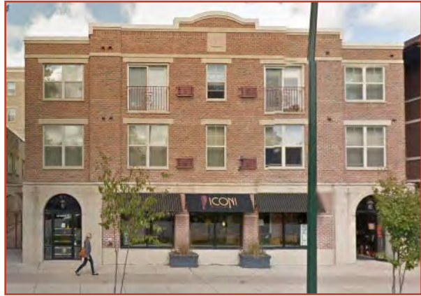
This building has architectural details that break down the facade to human scale and establish vertical proportions along a wide facade.
