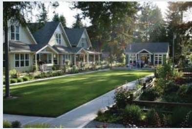
A bungalow court consists of a series of small, detached structures (500-800 square foot per unit), providing multiple units arranged around a shared court. Generally the homes are individually owned with the land under shared ownership.
