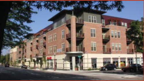
Various techniques in use to break down the apparent mass of a large building, including canopies, recessed decks, recessed top story, and variations in materials and wall plane.
