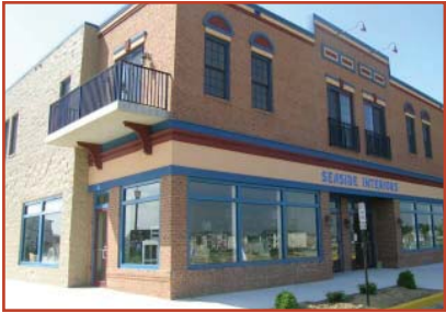
This example shows the use of a recessed entry to identify its location, and changes in material and wall plane to break up the side facade.
