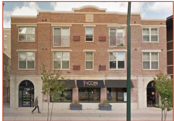
This building has architectural details that break down the facade to human scale and establish vertical proportions along a wide facade.
