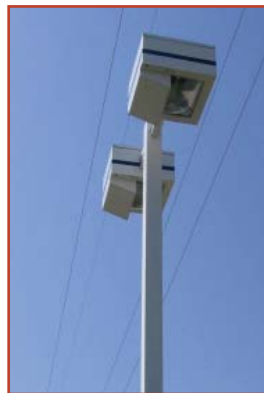
An example of a shielded light fixture that cuts down on light trespass.
