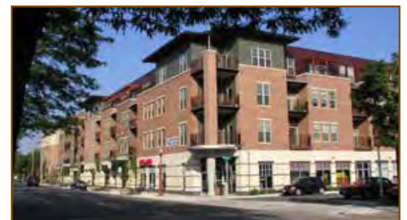
Various techniques in use to break down the apparent mass of a large building, including canopies, recessed decks, recessed top story, and variations in materials and wall plane.
