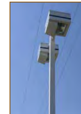
An example of a shielded light fixture that cuts down on light trespass.
