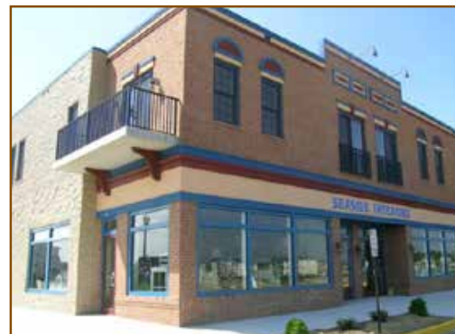
This example shows the use of a recessed entry to identify its location, and changes in material and wall plane to break up the side facade.
