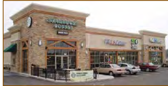
This building has architectural details that break down the facade to human scale and establish vertical proportions along a wide facade.
